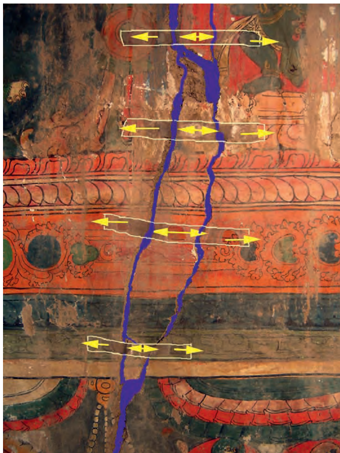
FIGURE 3 Portion of treated painting with schematic detail showing the location of mesh strips (yellow outline) used to secure plaster on either side of the cracks (blue). Arrows indicate adhesion points and the direction of forces that hold fragmented plaster in place.
