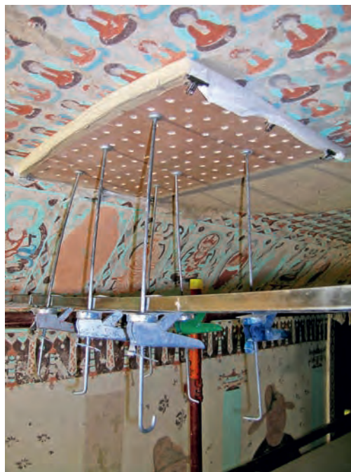
FIGURE 5 A customized press placed against treated plaster for support and to absorb moisture released from the grout. Photo: S. Rickerby
