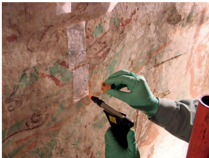
FIGURE 2 Salts being removed with the Preservation Pencil.
