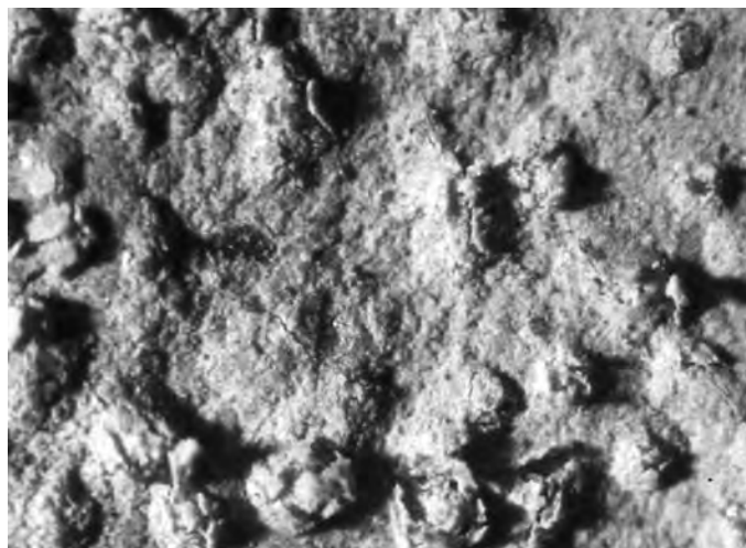
FIGURE 8 Salt eruption on the unpainted clay plaster.
