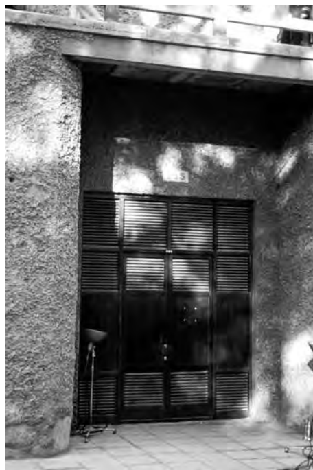
FIGURE 7 Exterior of cave 85 with door closed. A management decision was made to control relative humidity by keeping the cave closed during periods of rain when ambient relative humidity can rise to 75 to 80 percent.
