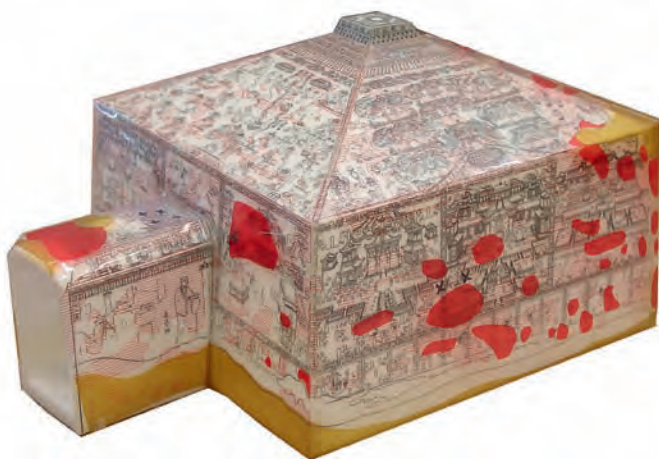
FIGURE 9 Scale model (1:35) of cave 85 with condition overlaid to show the distribution of deterioration.
