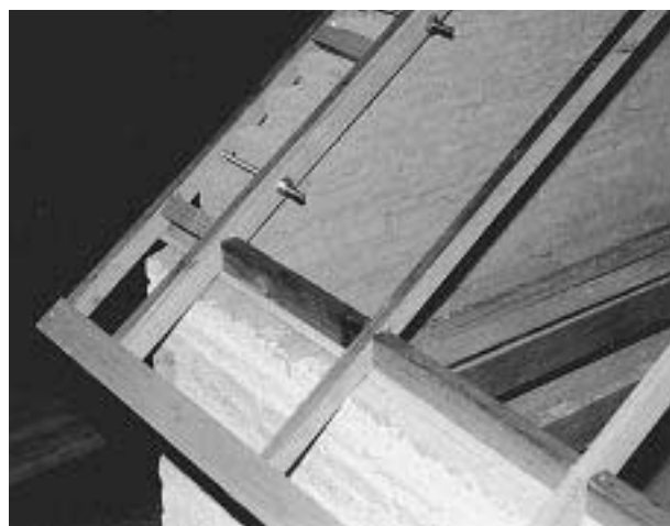
Figure 5.5 Blocking between roof rafters screwed to sill plate, used on models 8 and 9.
