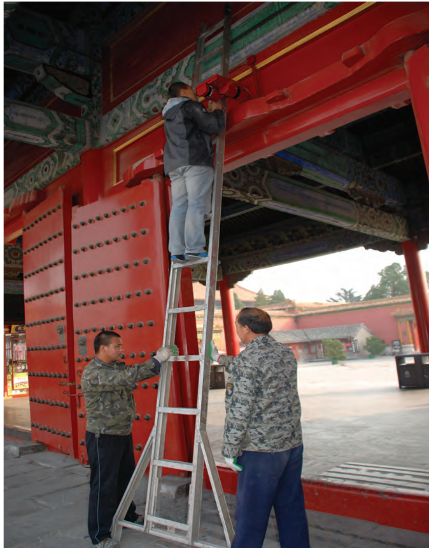
Figure 5. Installing visitor monitoring system in 2013.
