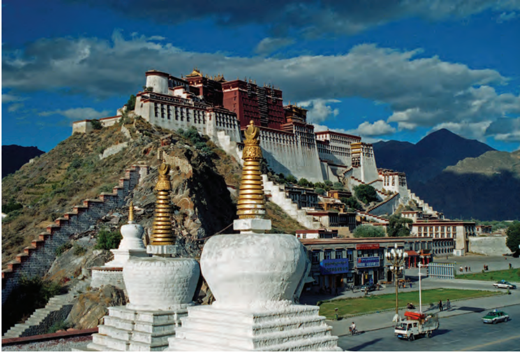
Fig. 1. General view of the Potala Palace.
